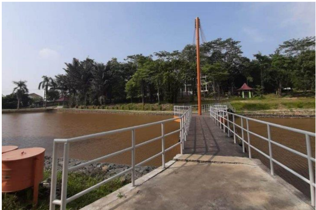
Example of Conventional Sewage Disposal Universitas Jambi (Septictank and Natural ponds)
